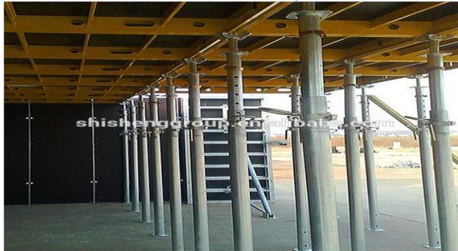
Figure:- 1.3 Hydraulic Props
